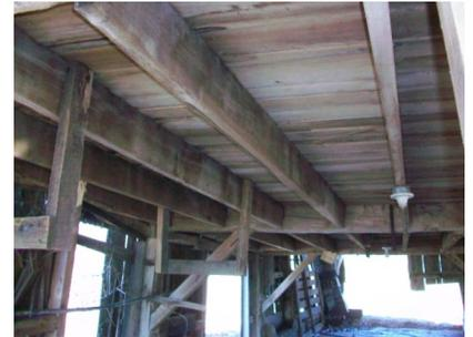
Cherry roof and floor boards lay across pit-sawn rafters and floor joists.
